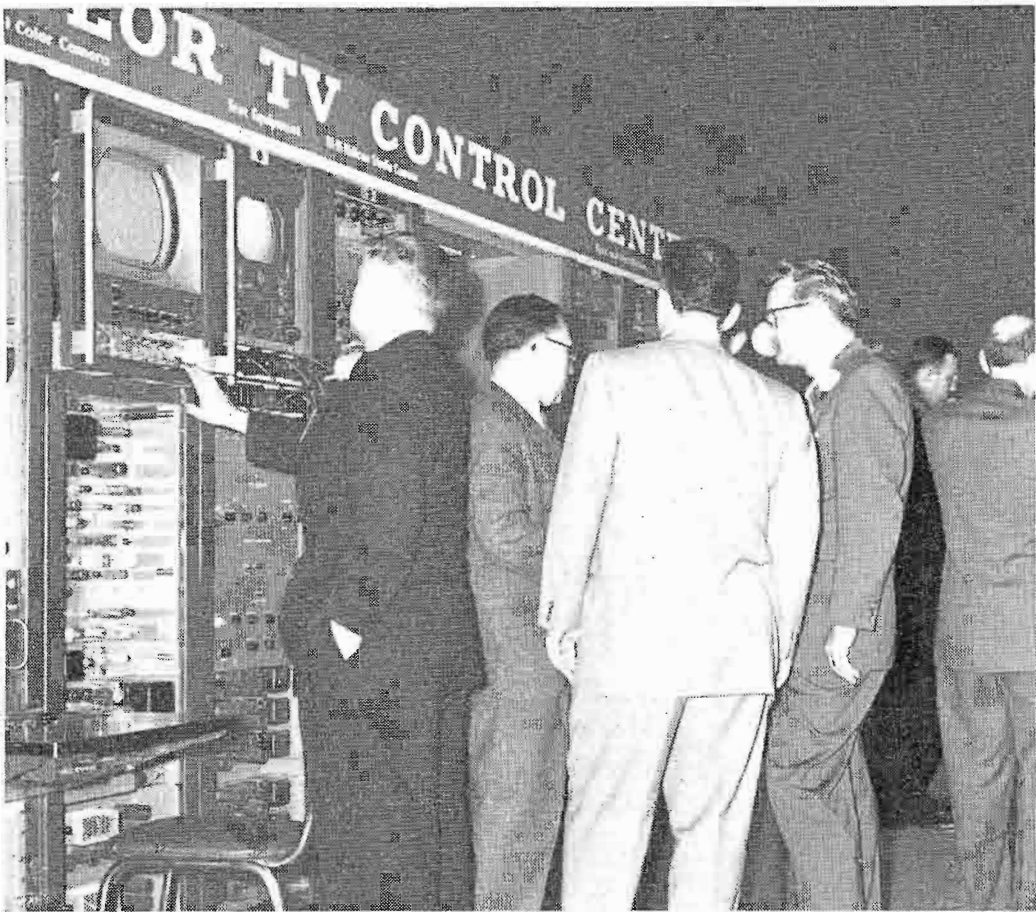
FIG. 4. Rack equipments for all operating displays were housed at the Color TV Control Center. This featured rack-mounted control desks for both TK-15 and TK-41 cameras.
